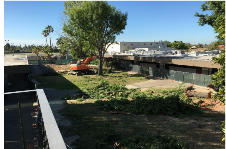
Science Courtyard Beginning Demolition
