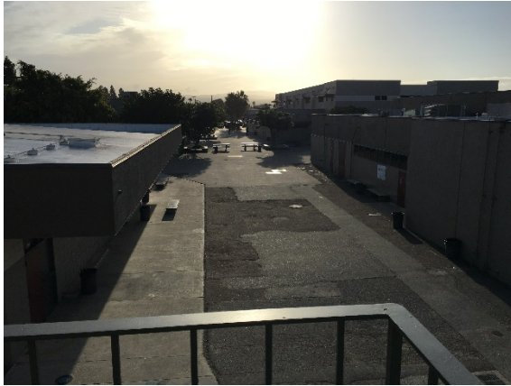
Original Entry Walkway
