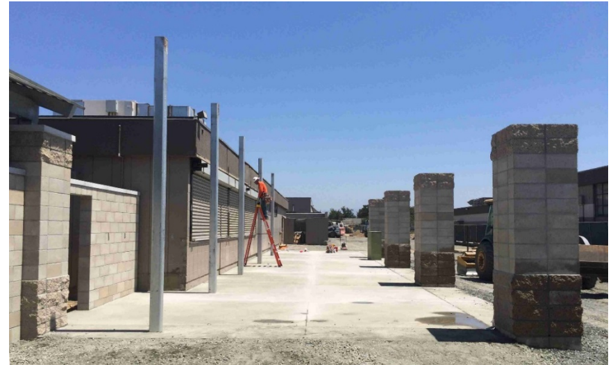
Custom Canopies Under Construction at Lunch Area
