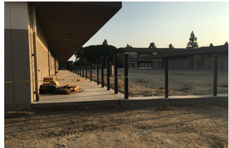
Science Courtyard with New Fence Posts
