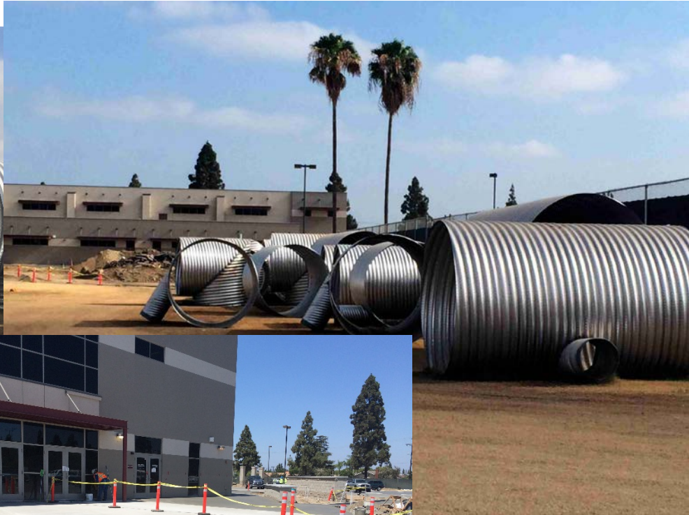
Detention Tank Piping
