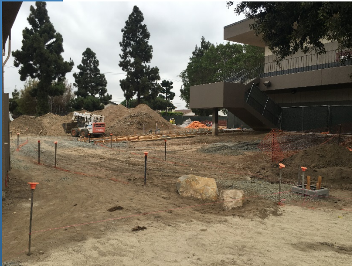
Phase A1 Courtyard Under Construction
